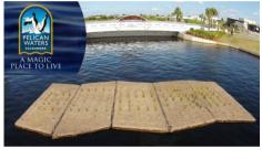
Through a collaboration involving the SWRG, Pelican Waters, Covey Associates, and SPEL Environmental, three Constructed Floating Wetlands (CFWs) are being fine-tuned at waterways within the residential estate of Pelican Waters.
